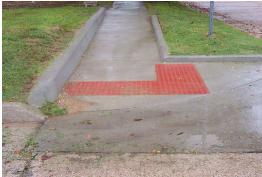
Good Condition: James and Sycamore streets
