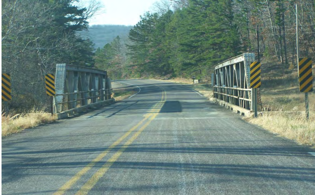
Image 3-1 Bridge over McGee Creek in Wayne County
