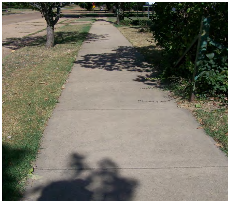
Good Condition: Fir Street
