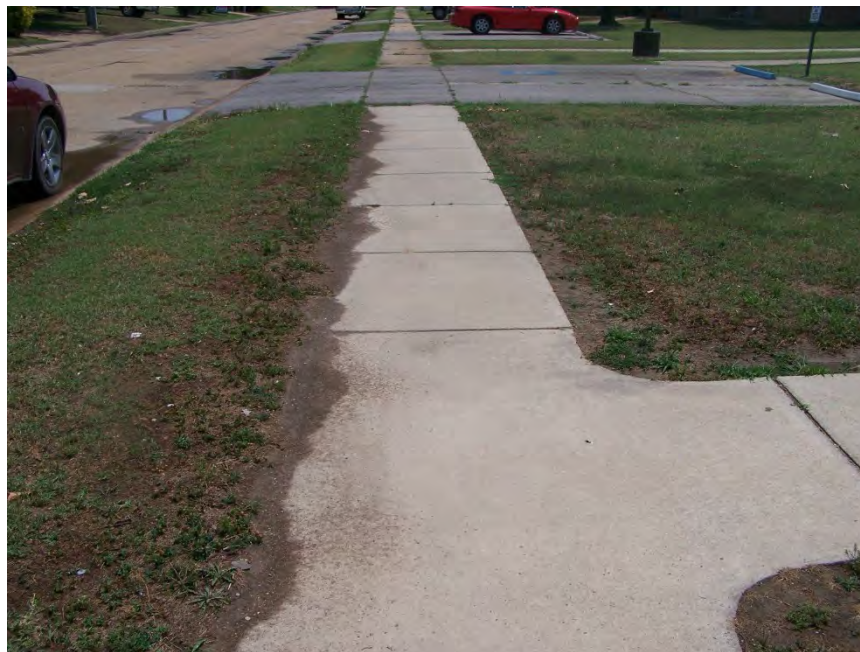
Good Condition: Tennessee St. facing south
