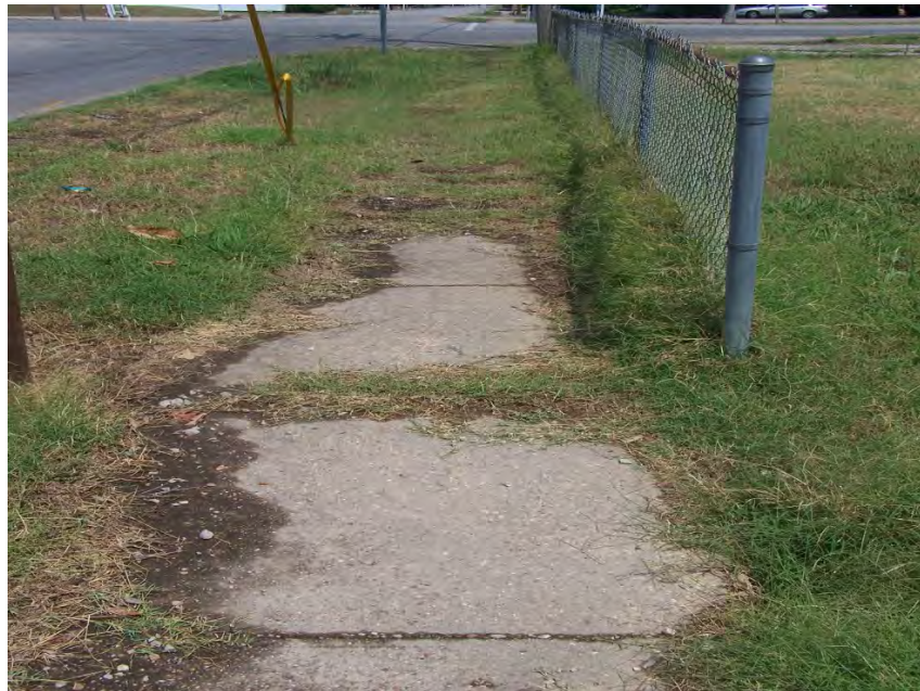
Poor Condition: Victor and Ditch Road facing east
