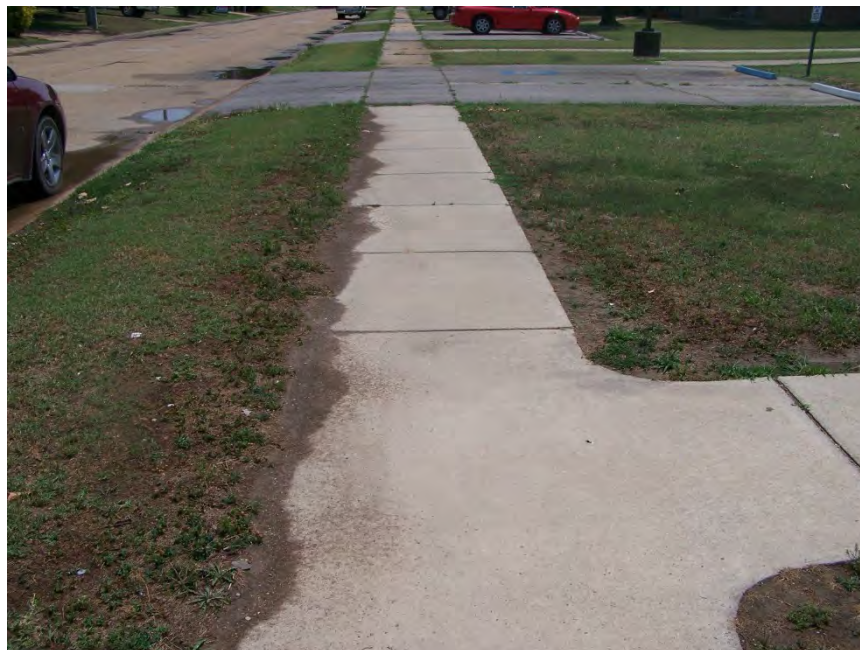
Good Condition: Tennessee St. facing south
