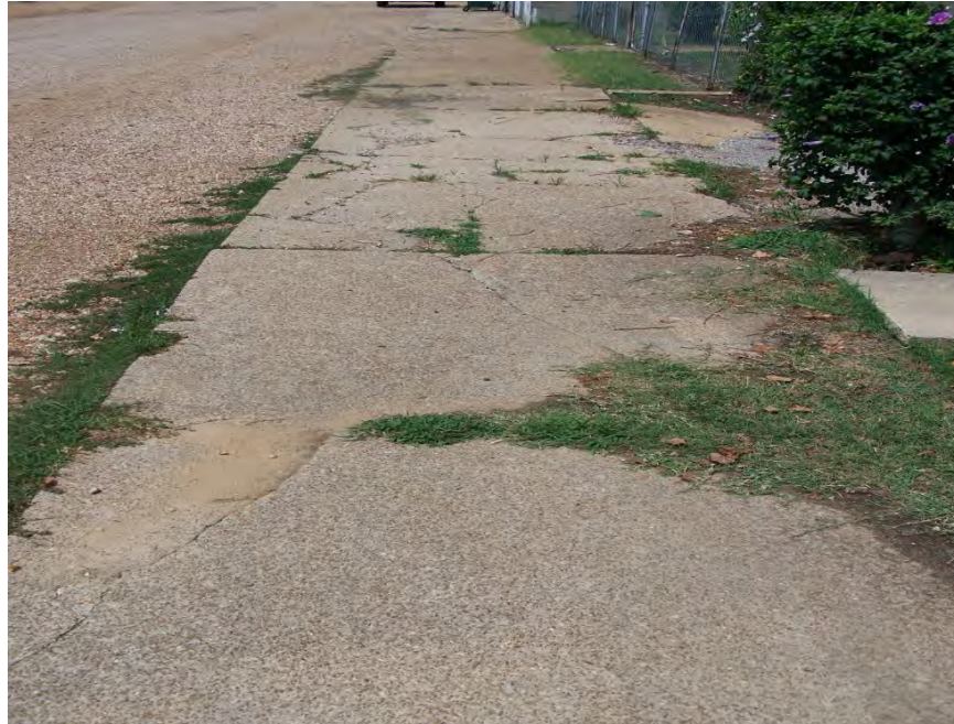
Fair Condition: Riverview facing north
