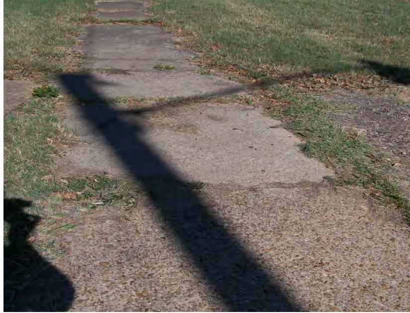
Fair Condition: Green and Forth Street facing west
