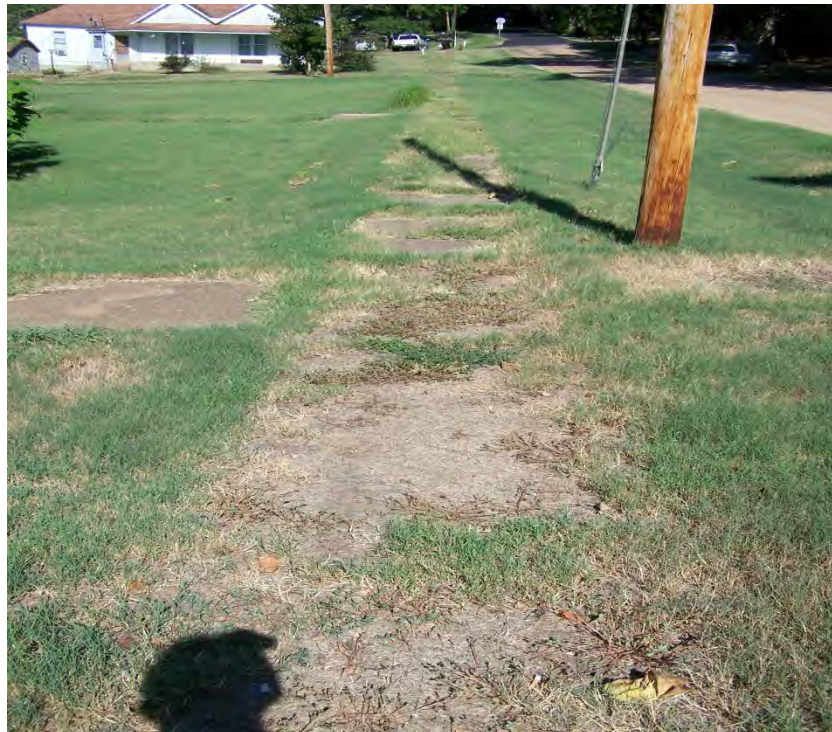
Poor Condition: Green Street facing west
