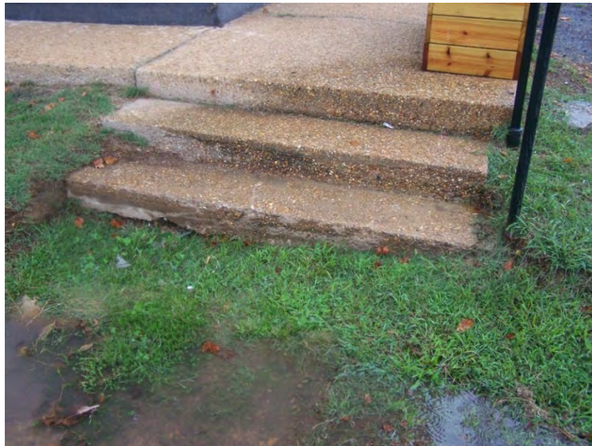
Poor Condition: Main Street facing south
