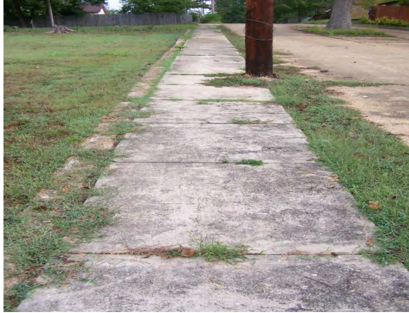
Fair Condition: East on Spring
