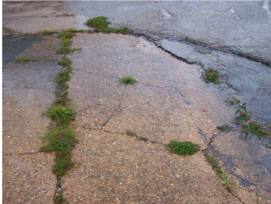
Fair Condition: Main Street facing north
