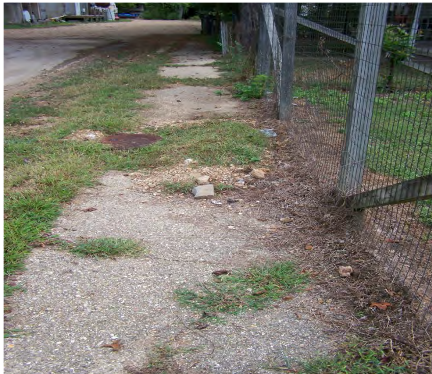
Poor Condition: Main Street North of Maple
